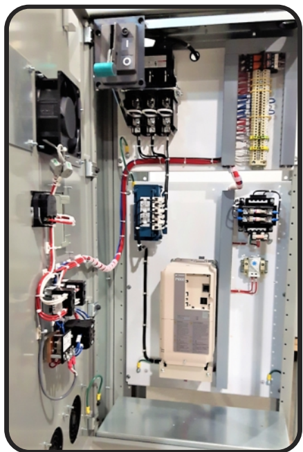
Layout of 25HP VFD panel
