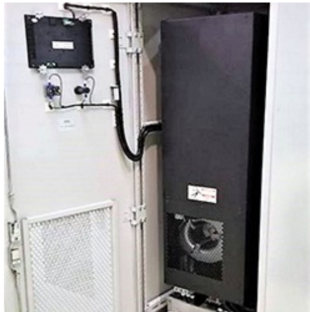
Figure 4: Internal APF layout with fan at the bottom
